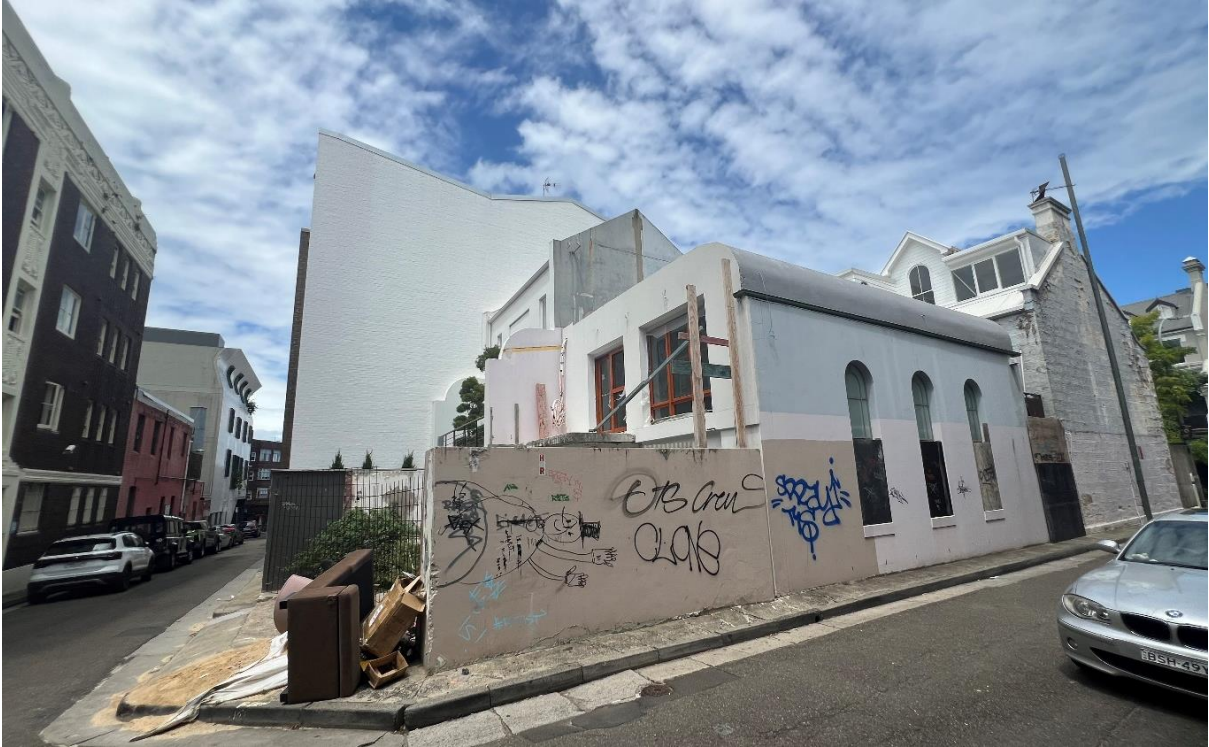
Figure 7: Residential terrace (under construction) on the opposite side of Kellett Way
